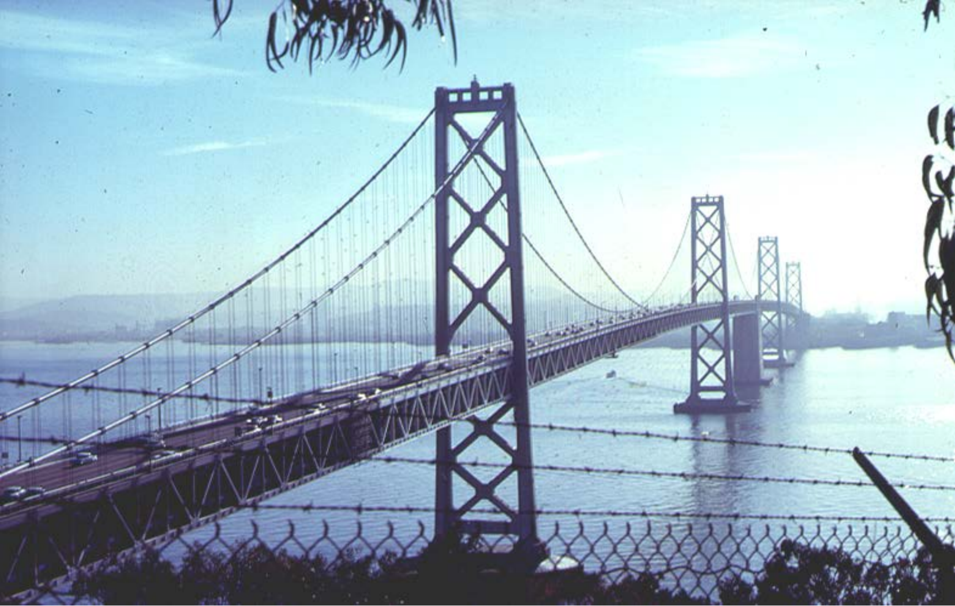
San Francisco-Oakland Bay Bridge (1936)
