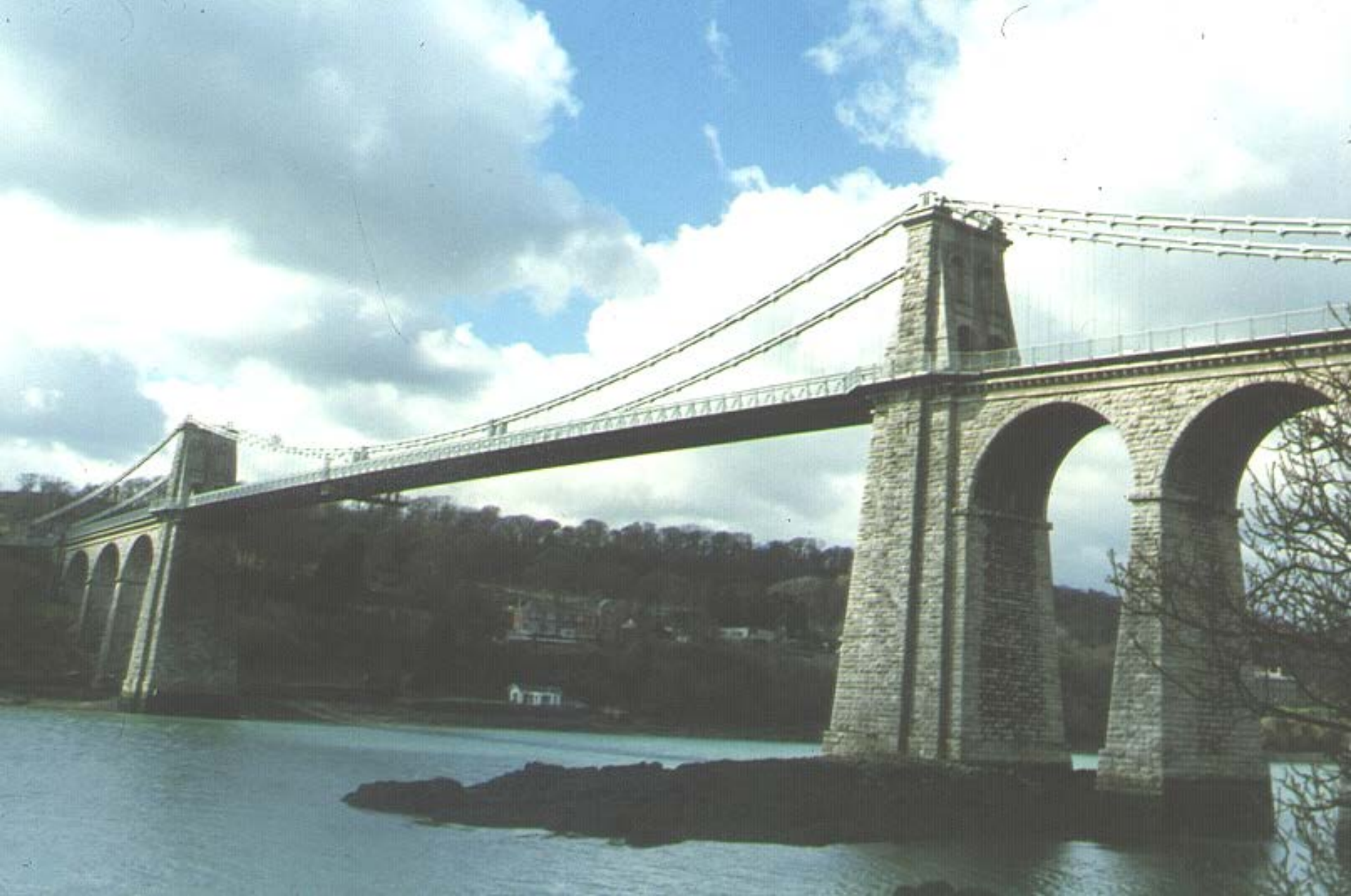
Menai Bridge 1826 (British) 176 m
