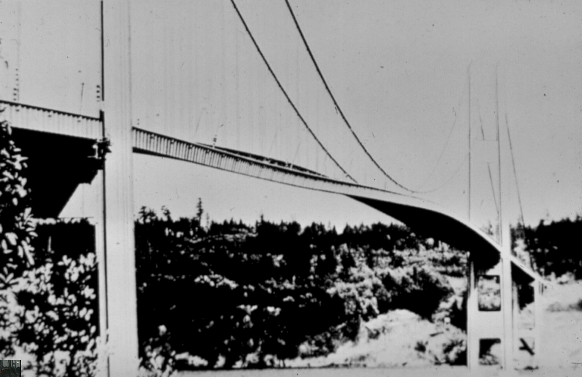
Tacoma Narrows Bridge (1940) 855m
